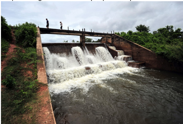
Figure 28. Spillway at Houay Siet Dam, with simple pool fishway on the right
