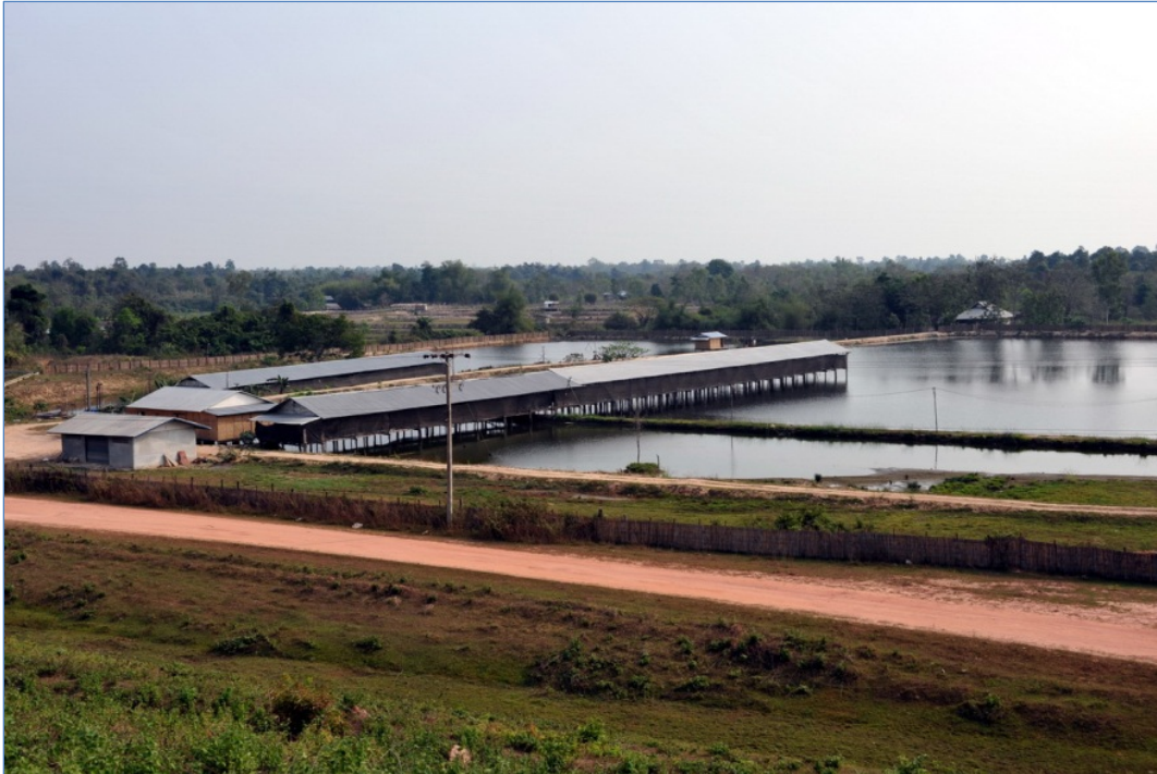
Figure 13. Integrated chicken-fish farm on the downstream side of Nam Houm Dam wall
